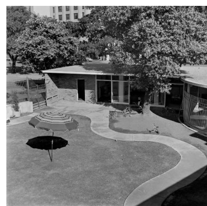
42 Playground and creche associated with the Hyde Park women's amenities centre.
