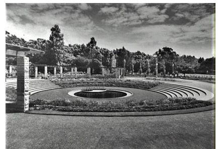
73 Sandringham Gardens as initially conceived, 1952. Source: CSA Unique ID A-00014658
