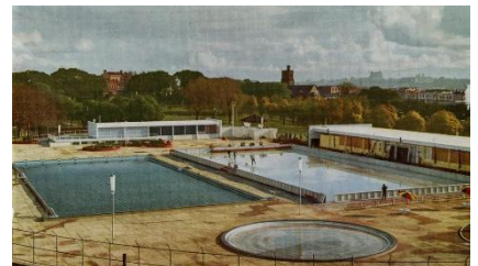
28 Swimming pool complex in Prince Alfred Park. Source: CSA Unique ID A-00008445.
