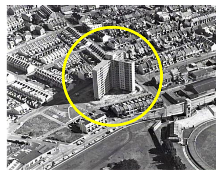
21 John Byrne Court in Glebe, completed in 1961. Source: CSA UID A- 00012502.
