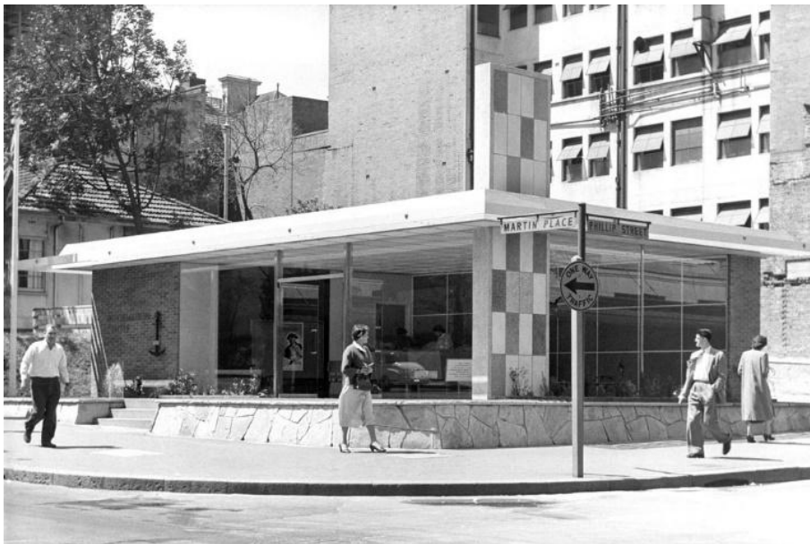
60 The stylish Modernist Information Bureau at the eastern end of Martin Place, constructed just prior to the Melbourne Olympic Games in 1956.
