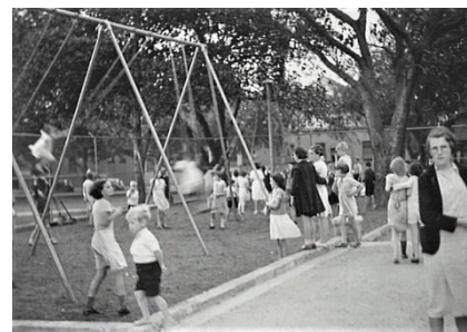
31 The girls’ playground at the time of its opening in December 1935. Source: CSA Unique ID A-00055480.
